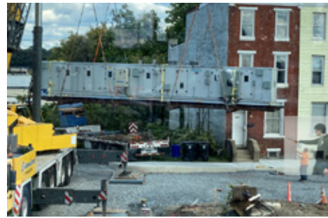
A construction worker helps lift one of the Munter Unit machines into the new PA State Archives building. Courtesy of PHMC, 2022.
