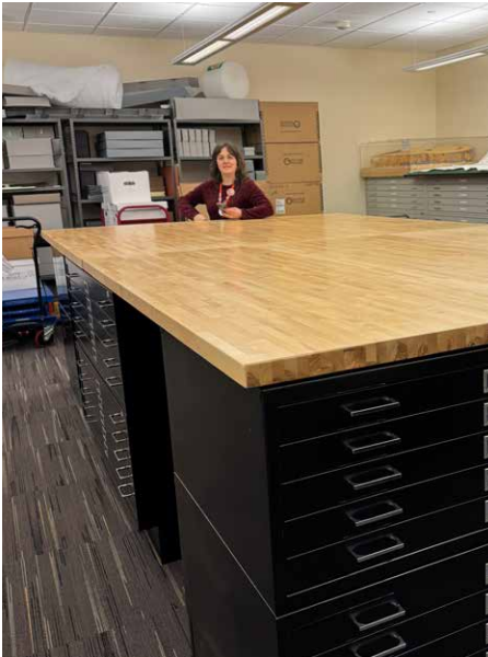
TOP: The map case base that was built prior to the maple butcher block installation.
