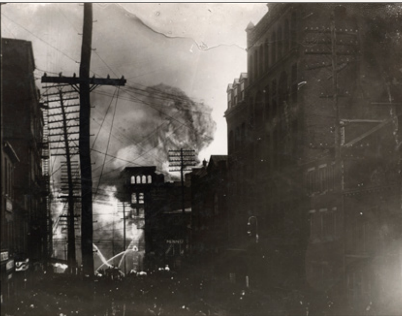
John E. Hurst and Company Building Engulfed in Flame Soon after Start of Fire. 1904. Enoch Pratt Free Library. J. H. Schaefer and Son.
